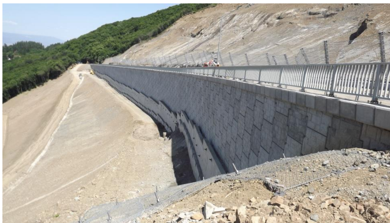
Fig. 2. A newly built load-bearing wall and a highway located on it.
