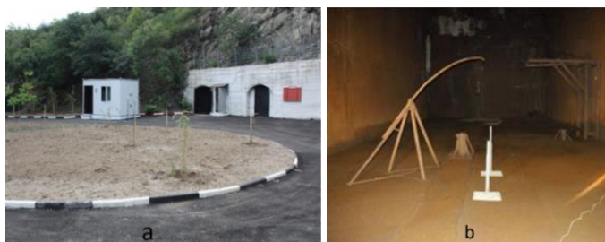
Fig. 1 The portal of the underground tunnel system (a) The blasting camera (b)
